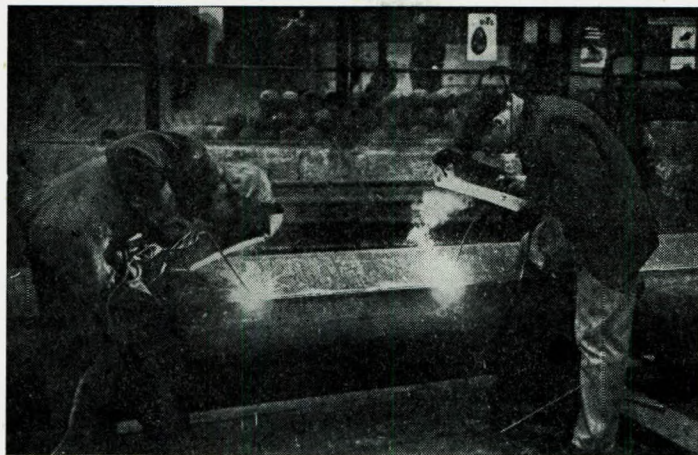
FIG. 19.—Welders at work on an ash shoot for a new vessel in a modern shipyard. Welding means "clean" construction, due to the elimination of angle brackets and plates.
