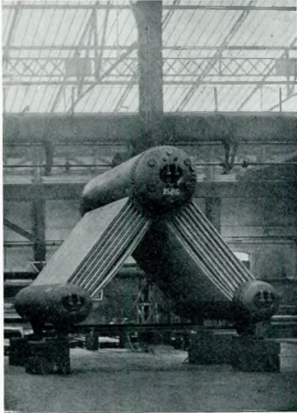
FIG. 14.—Yarrow boiler without superheater.
