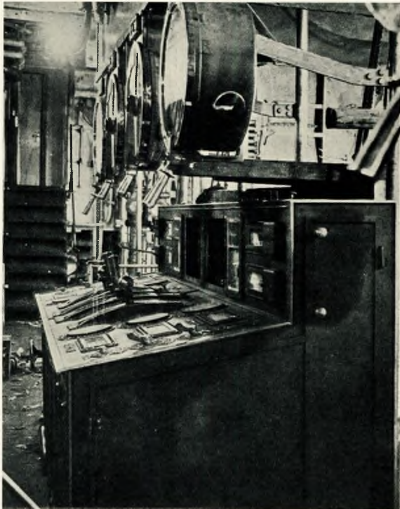
FIG. 15.—View of control desk installed on board.
