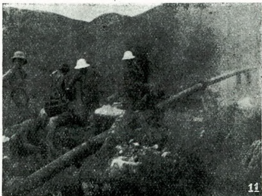
The Fitters at Work, and a View of the Steep Mountains.
