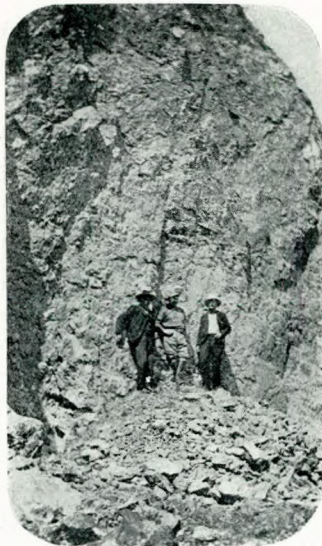
5.—Caved in workings, Waterson Mine, Ocampo.
