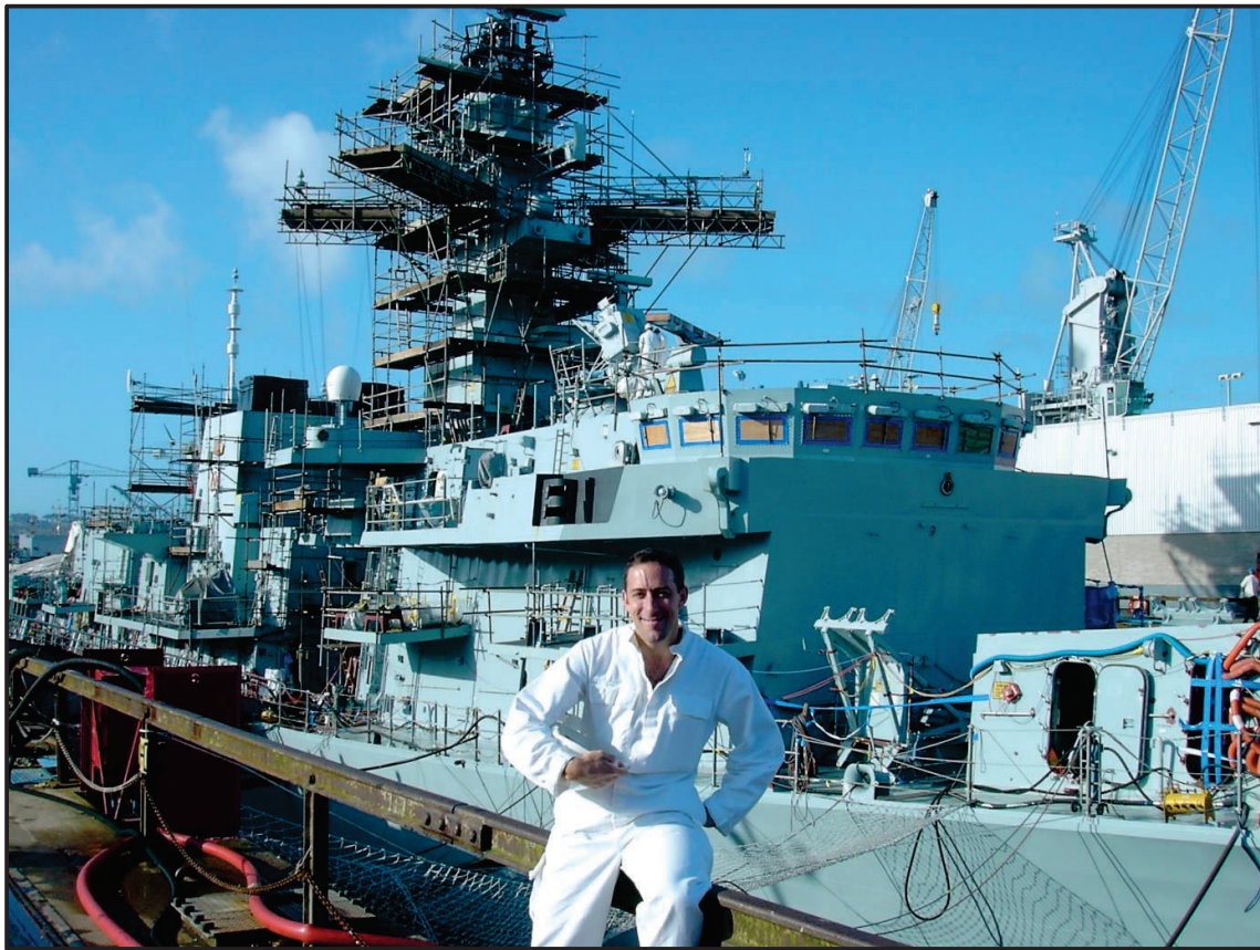
Figure 5: HMAS LANCLOVELY in Build
