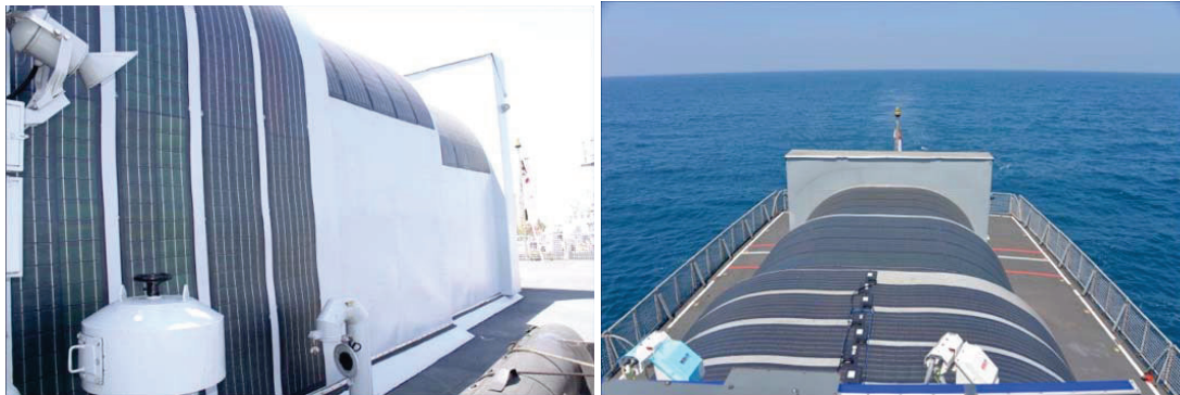
Figure 8: Solar Panels Installed on the Hello Hanger of INS Sarvekshak
