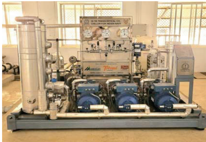
Figure 11: AC plant with CO 2 as a refrigerant #
