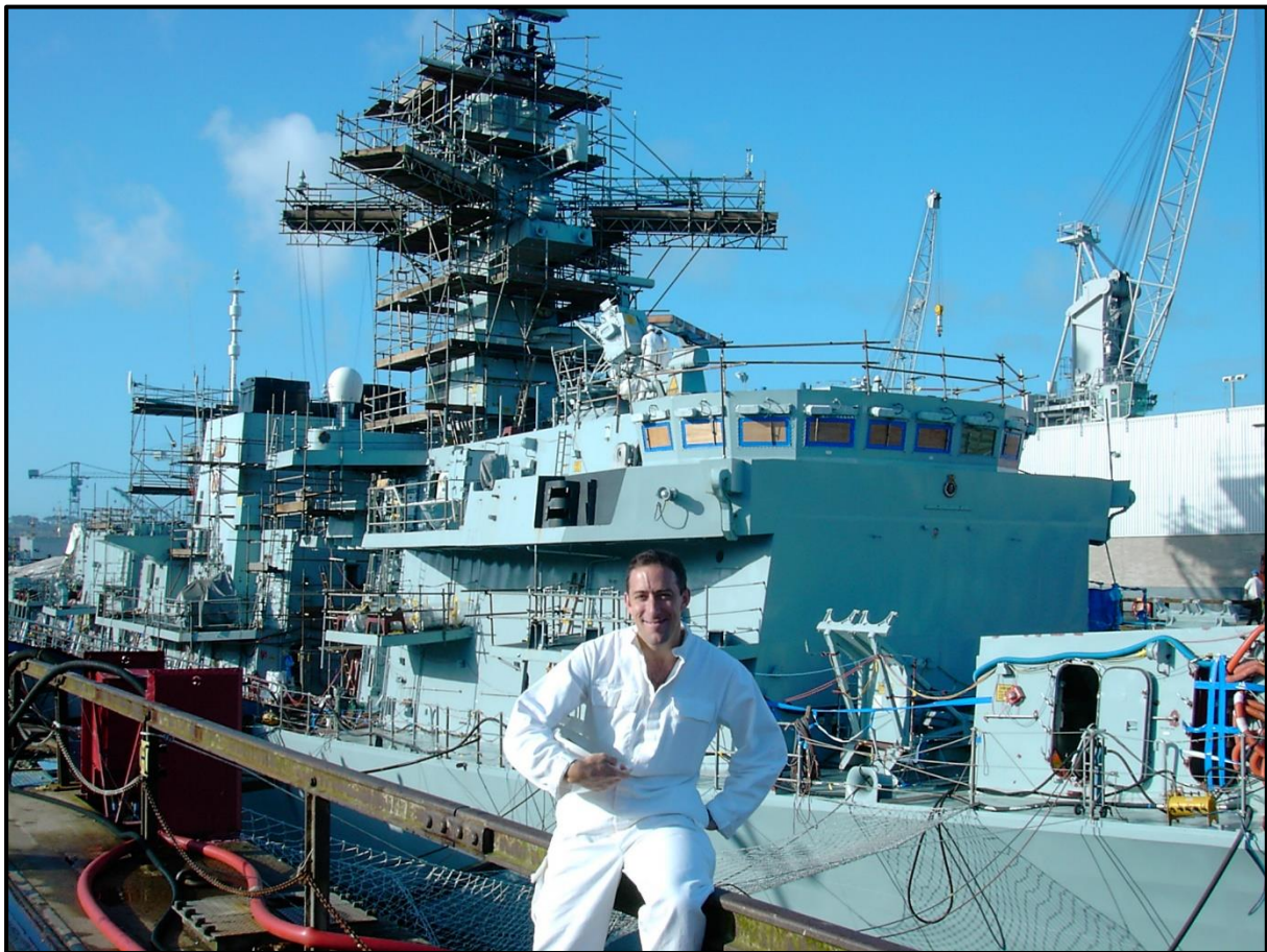
Figure 5: HMAS LANCLOVELY in Build
