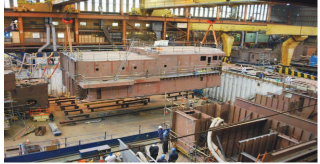
Fig 6: Build yard for the Irish OPV project, UK (courtesy of Babcock)
