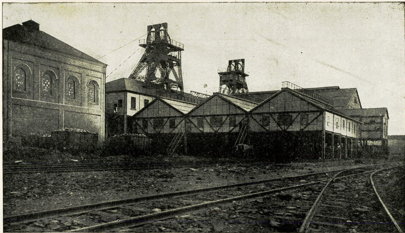
478A.—Modern steel headgear and screening plant, Easington Colliery, Co. Durham. Head Wrightson and Co.
