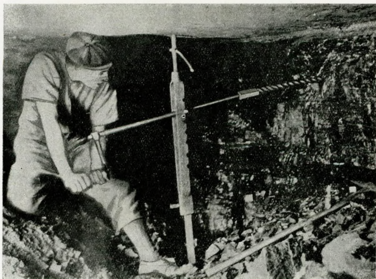
Copyright. With permission of Ashington Coal Co. 14.—Boring shothole by hand, Ashington Colliery, Northumberland.
