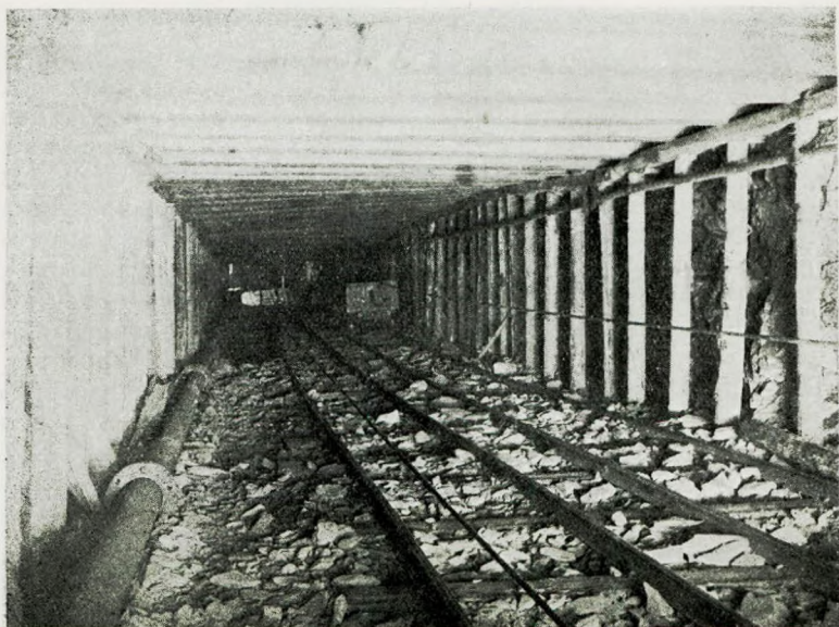
Copyright. With permission of Ashington Coal Co. 7A.—Rolley way timbering, Ashington Colliery, Northumberland.
