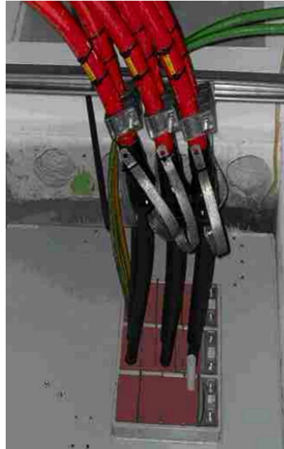
Figure 2-MV Cable Termination (1250 A 7.6 MW)
