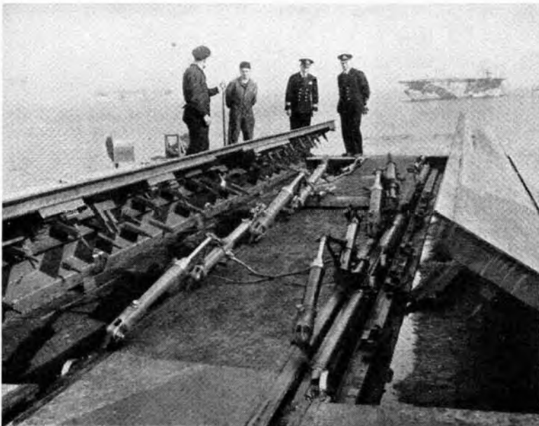
FIG. 14. T.T. Mk. III TROLLEY. STOWAGE COVERS OPENED
