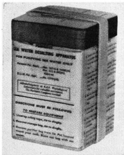
FIG. 1.— 4\frac{1}{2} PINT EQUIPMENT FOR BOMBER AIRCRAFT. WEIGHT 2 LBS.
