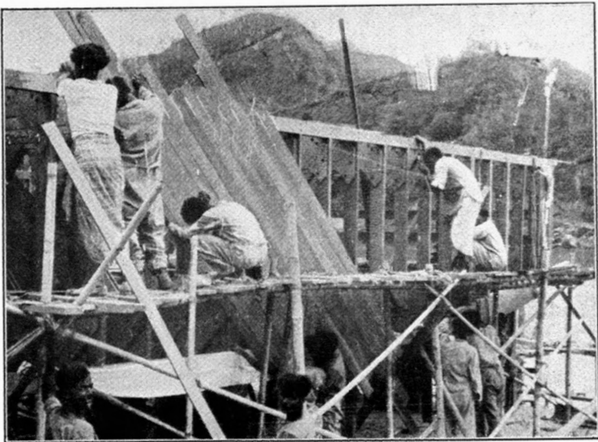
AT WORK ON THE SIDE PLANKING
