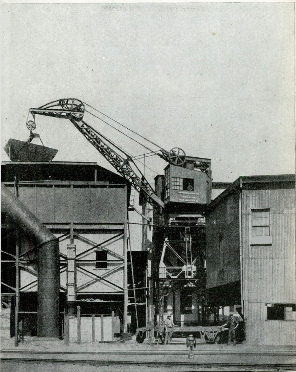
157B.—10-ton lever balanced luffing crane for power station, Brisbane Tramways Co.
