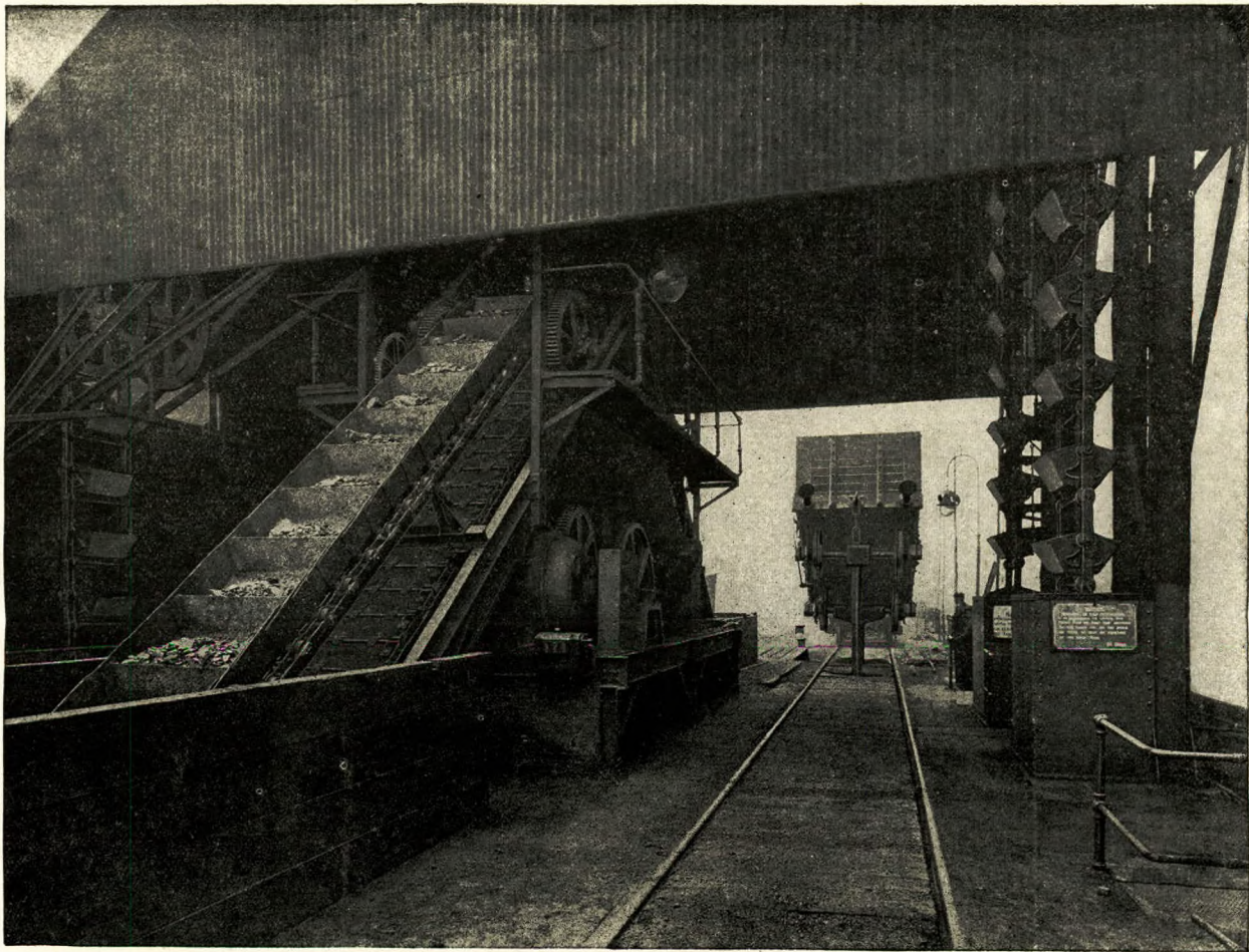
152A.—End door wagon tip and coal handling plant, Birmingham Corporation Gas Works, Saltley.
