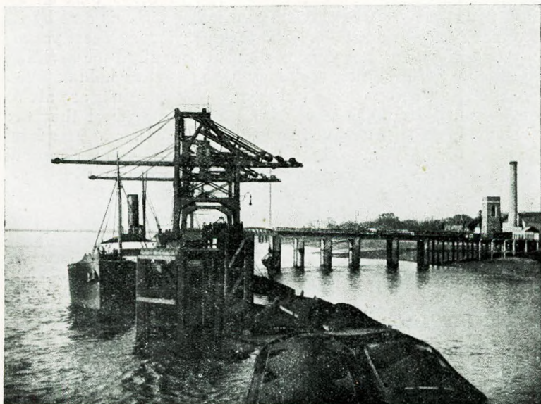
137.—Purfleet Pier, 1905, 2 cranes grab discharging inside pier.
