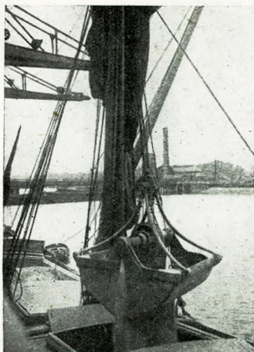
141.—Purfleet Pier, loading the forehold of a sailing barge with grabs.
