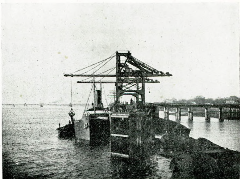
137A.—Purfleet Pier, 2 cranes grab discharging outside vessel.
