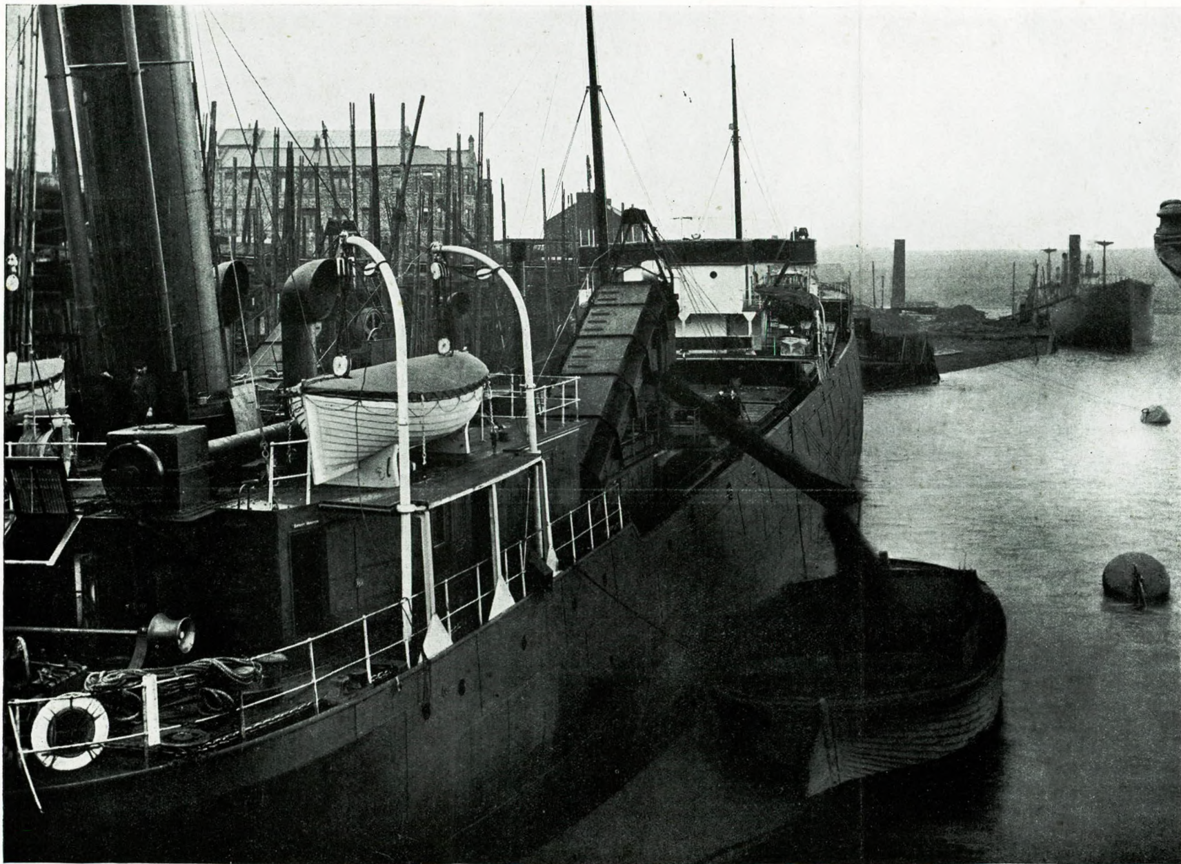
135A.—Doxford's self-discharging collier, "Herman Sauber," discharging 1,200 tons per hour.
