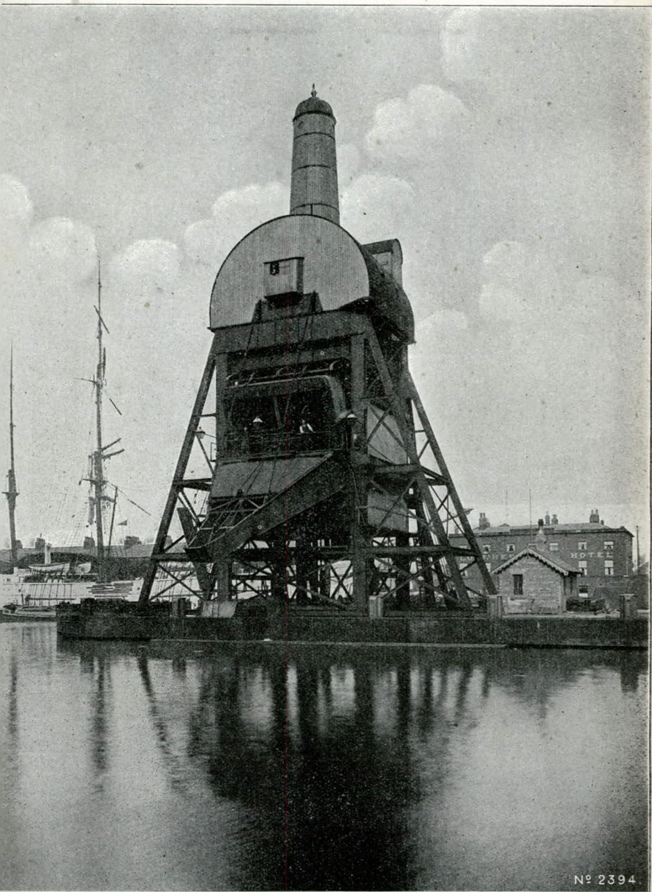
110.—Special hoist, Goole Docks. Armstrong Whitworth.
