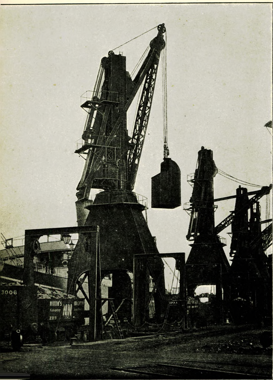
106.—Lewis Hunter hydraulic coal crane, by Sir W. G. Armstrong, Whitworth & Co.
