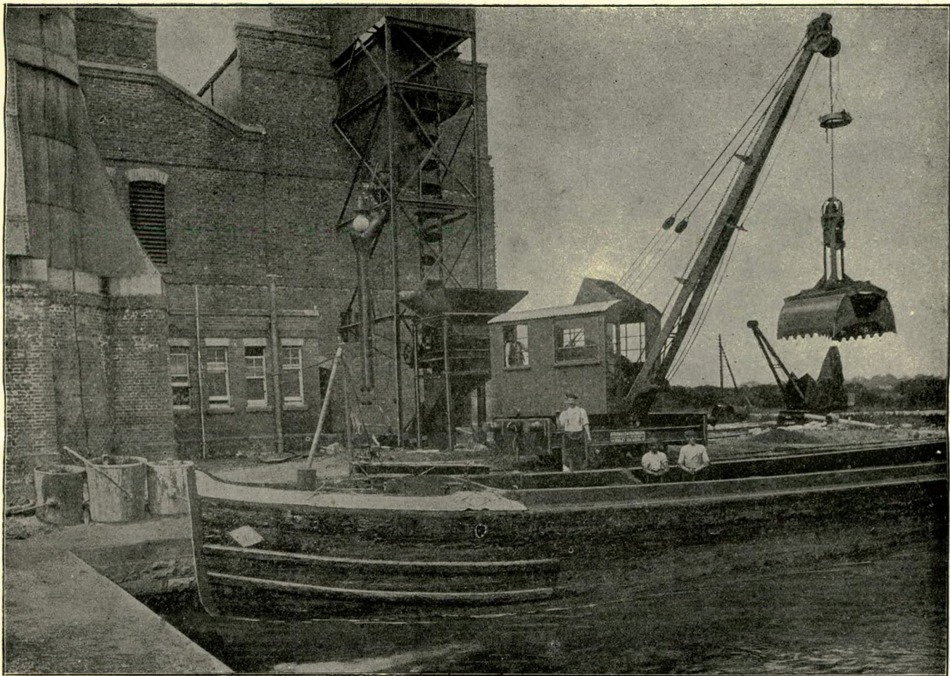
153A.—North Metropolitan Electric Supply Co., Brimsdown, conveyer and coal handling plant.
