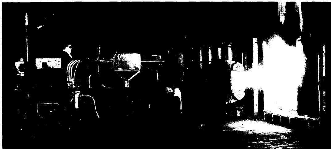
WELLMAN SMITH OWEN MOBILE FORGE MANIPULATOR WITH "V.S.G." EQUIPMENT
