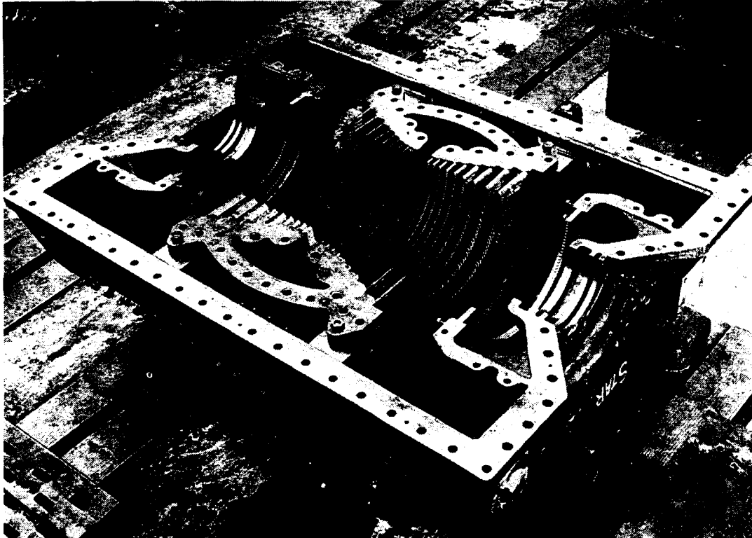
DOUBLE-FLOW L.P. REACTION CASING
