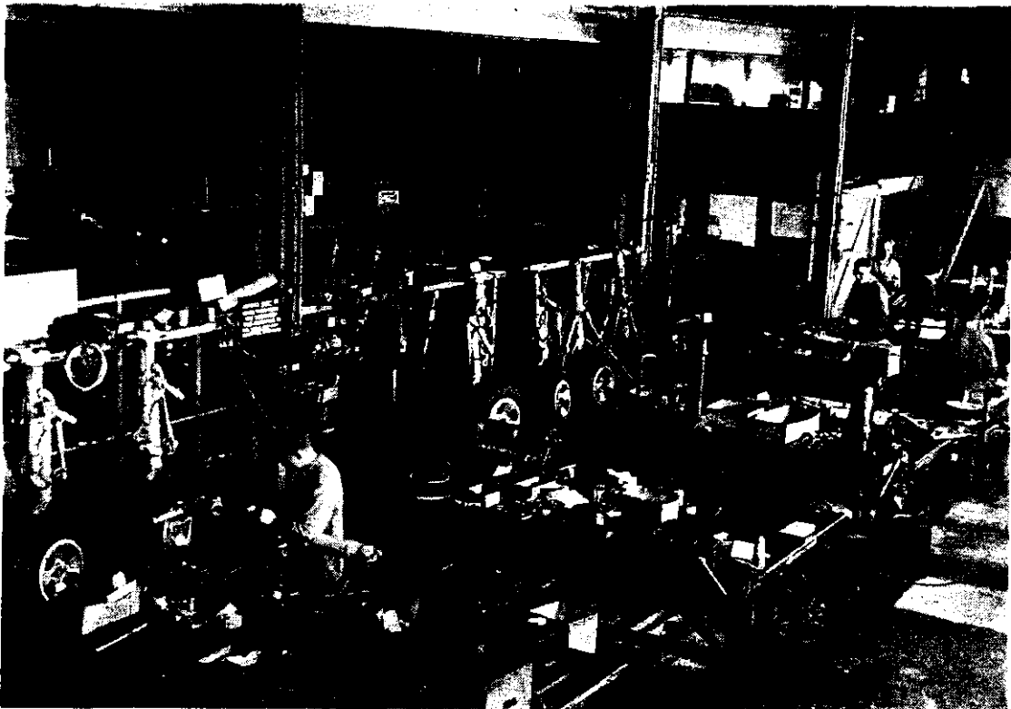
SECTION OF HYDRAULIC SHOP SHOWING RE-CONDITIONED UNDERCARRIAGE PARTS
