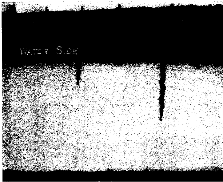
FIG. 17—SECTION THROUGH WALL OF A30 SHOWING TRANSVERSE CRACKS
