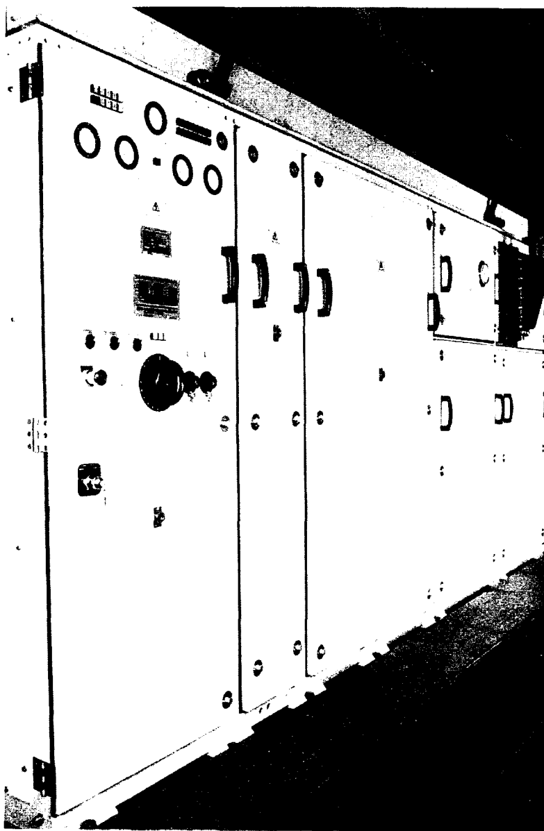
FIG. 5—THE REGULATOR AND CONVERTER UNIT, SHOWING THE LOCAL CONTROL PANEL IN THE FOREGROUND
