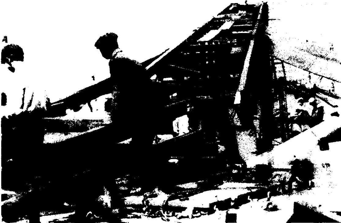
FIG. 19—THE EARLY CATAPULT INSTALLATION ON 'NORTH CAROLINA', 1916
