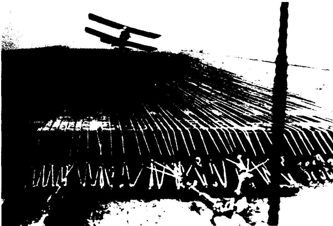
FIG. 10—SUMMER 1918. A SOPWITH PUP CAUGHT UP IN THE TURBULENCE OVER 'FURIOUS'S' AFTER DECK. THE EARLY INSTALLATION OF AXIAL HOLD-DOWN WIRES CAN CLEARLY BE SEEN
