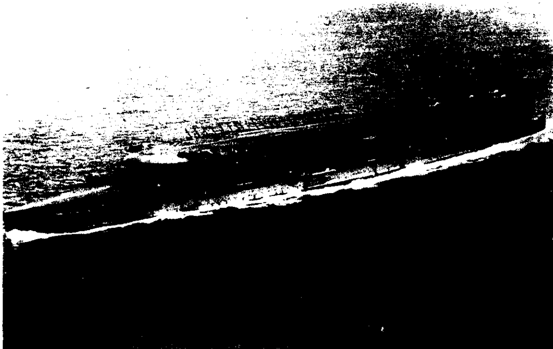
FIG. 15—'FURIOUS', AFTER HER MAJOR REBUILD, NOW A FLUSH-DECK CARRIER OF THE 1930s. THE PALISADES, INSTALLED IN 1926, WERE TO PREVENT AIRCRAFT GOING OVER THE SIDE AFTER A BAD LANDING
