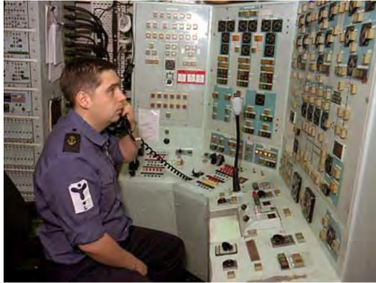
FIG.1 – TRADITIONAL CONTROL PANEL
