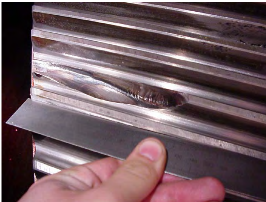
FIG.11 – HMS ILLUSTRIOUS ' MAINWHEEL FAILURE
