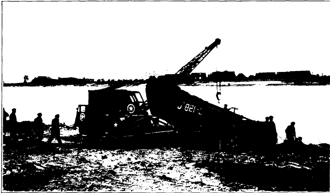
FIG. 2.—LANDING CRAFT BEING LAUNCHED INTO THE RHINE DOWN SPECIALLY PREPARED SLIPWAYS
