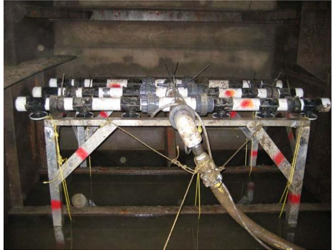
Photo 8 - Grid diffuser in tank
