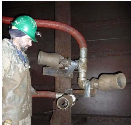
**Photo 5 - 45° nozzle setup (lower nozzle part of parallel setup)**
