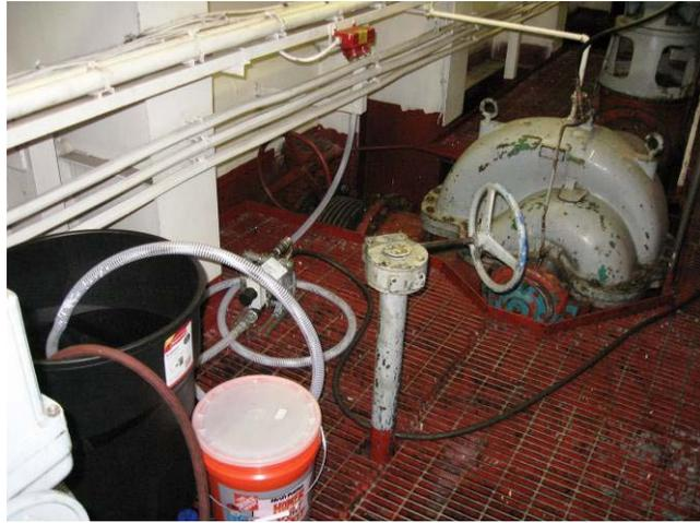
Photo 7 - Inline dosing setup
