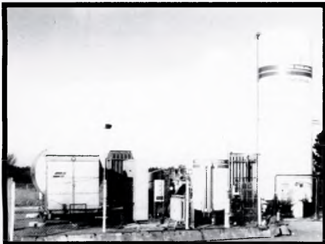
Fig 9: Gas supply unit, dominated by the large LNG tank
