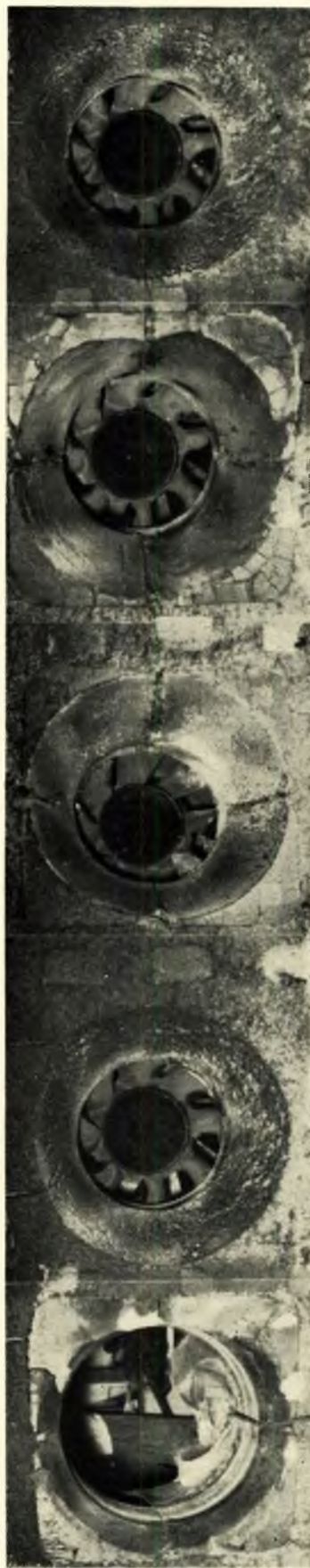
(b) Starboard aft boiler
