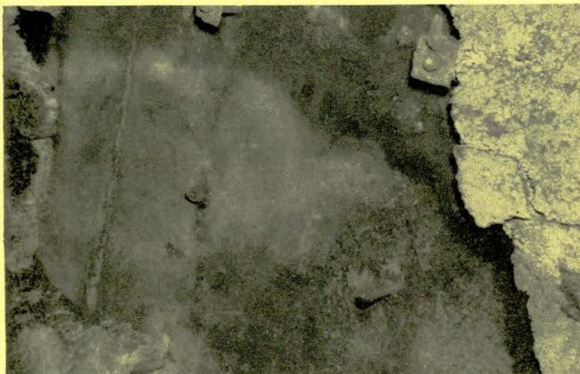
FIG. 18—Back wall of single-pass header type boiler stripped for replacement of rammed plastic lining (four years' service). Note burned-off anchor bolts
