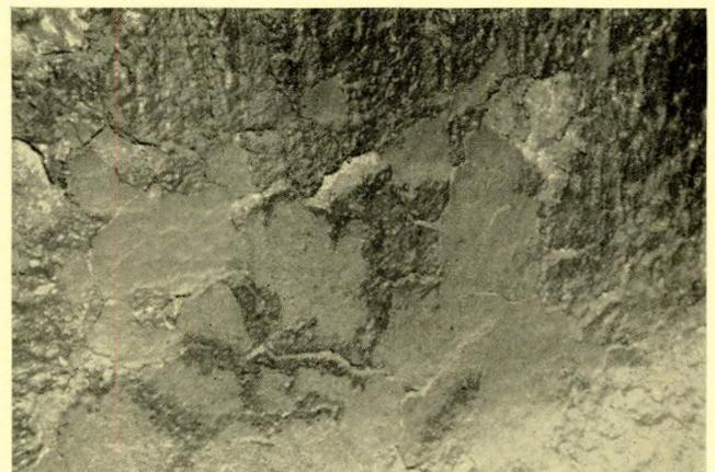
FIG. 17—Back wall of D-type boiler (four years' service)
