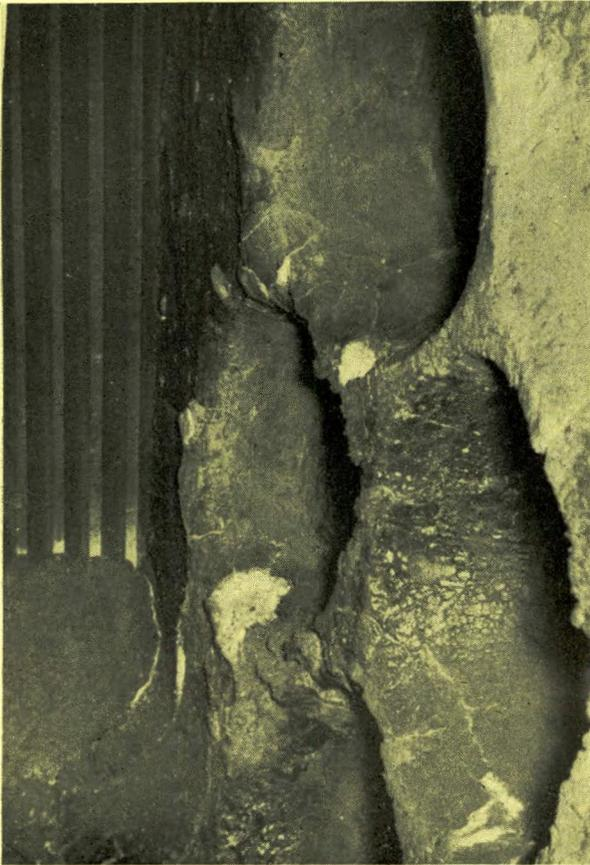
FIG. 25—Burner quarl section in a D-type boiler
