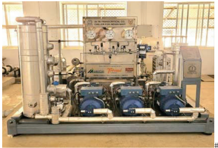
Figure 11: AC plant with CO 2 as a refrigerant
