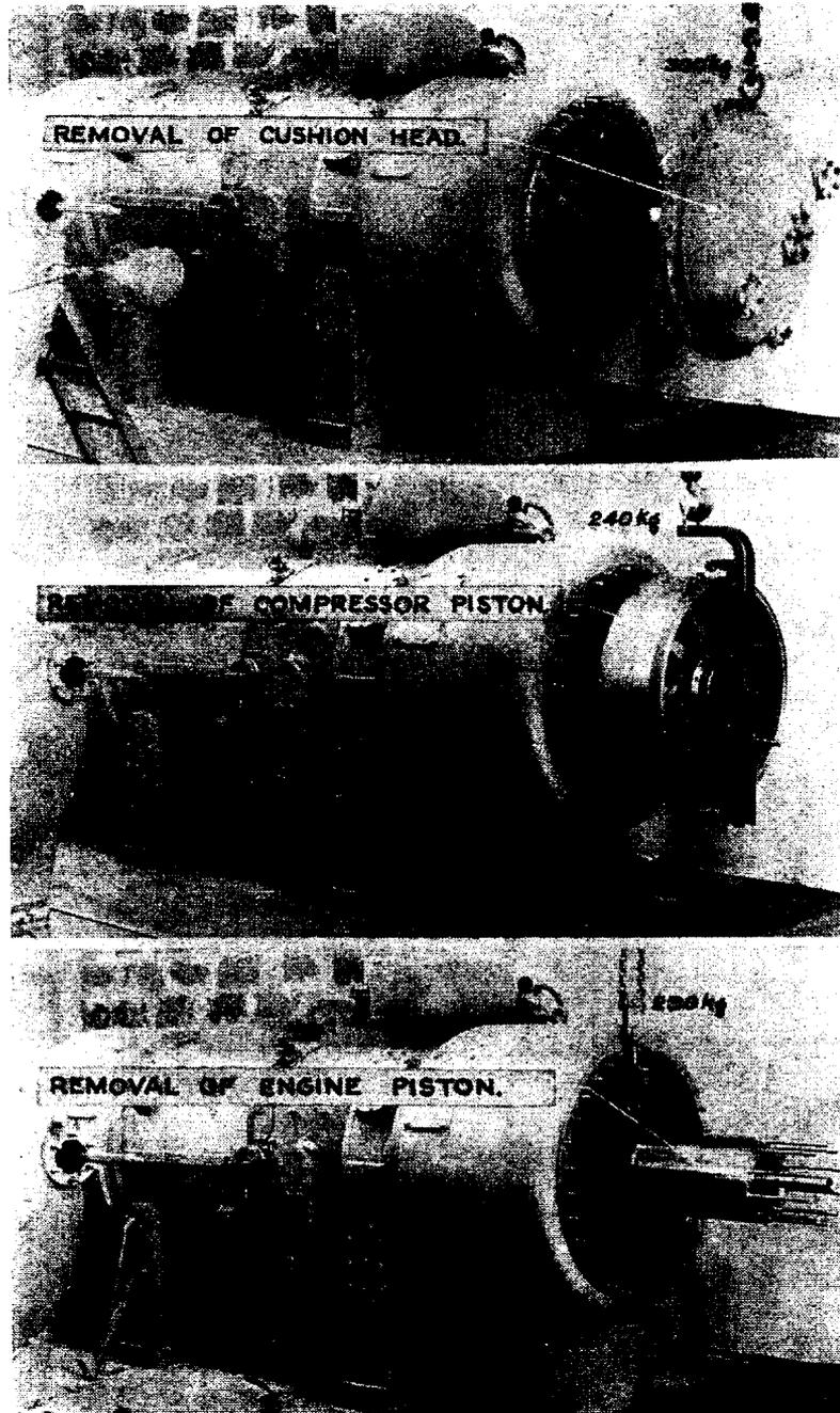
FIG. 5—DISMANTLING A G.S.-34 GAS GENERATOR
