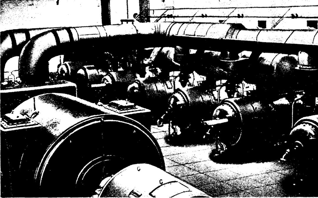
FIG. 4—PART OF A 6,000 kW. GENERATING PLANT AT CHERBOURG WHICH EMPLOYS EIGHT GASIFIERS
